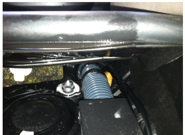
Picture 2A: View from the engine compartment
